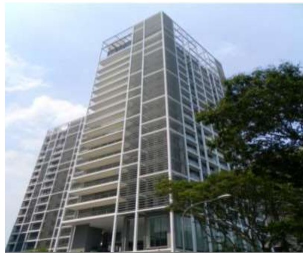
Urban Resort Condominium
