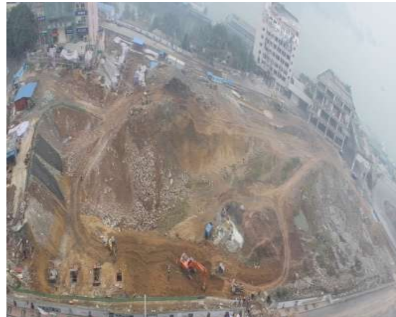
Excavation work under progress
