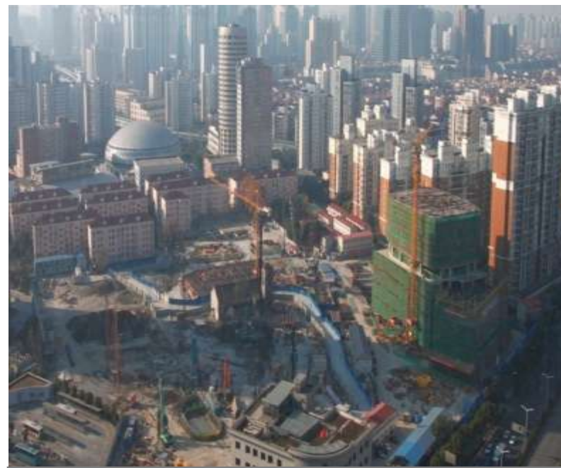
Aerial view: 19% completion
