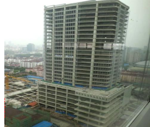
Structural completion for Tower 2
