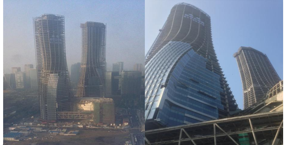
Curtain wall installation in progress
