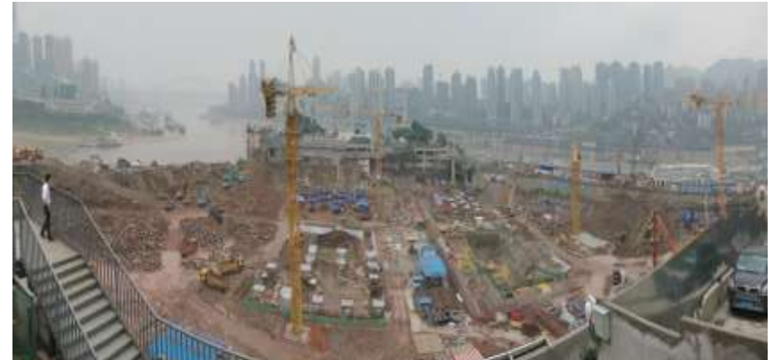
Obtained Planning Permit For Basement And Piling
