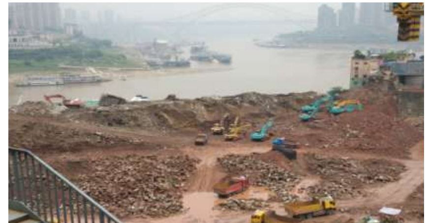
Demolition Of Harbour Office And Ramp Completed
