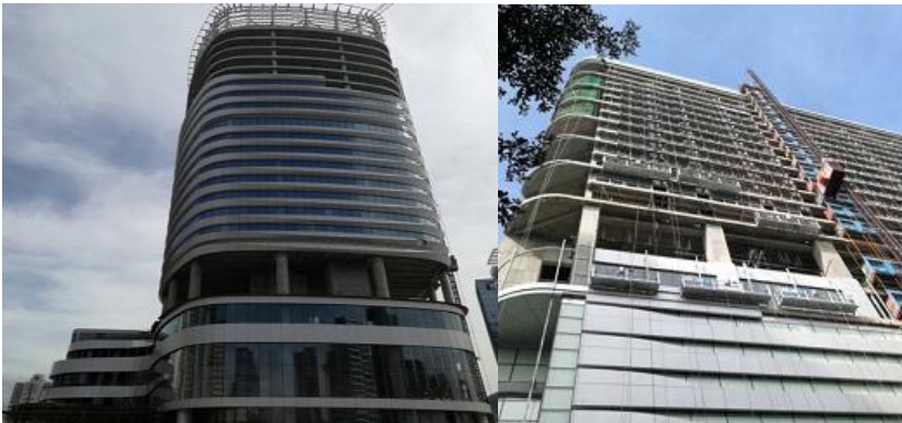
Curtain Wall Installation For Tower Podium
