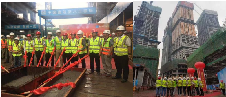
Topping Out Of Tower 3 (South)
