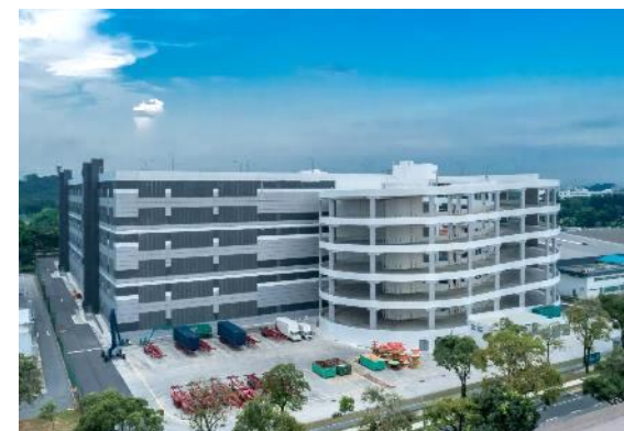
20 Tuas Avenue 1, Singapore
