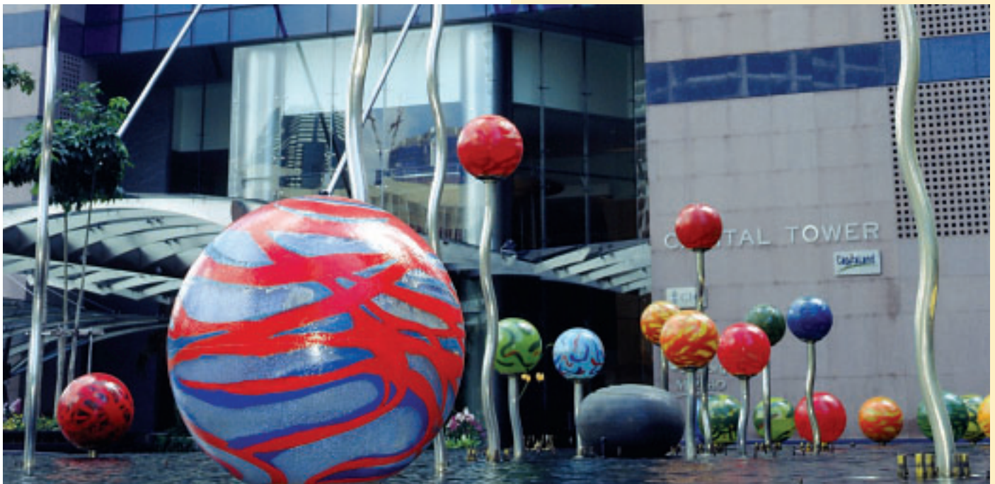
Capital Tower, Singapore, a landmark and award-winning property in the central business district.
