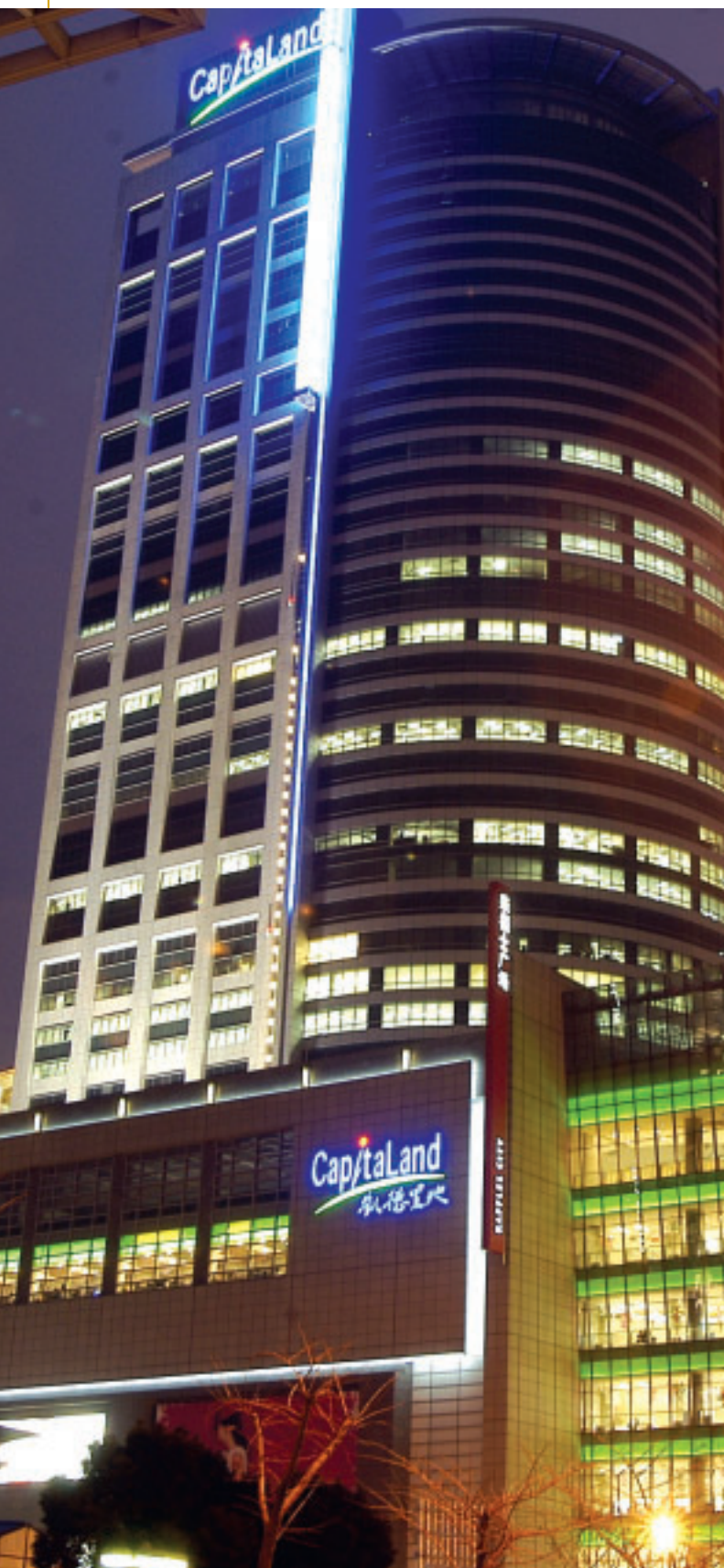
Raffles City Shanghai, a landmark building in China.
