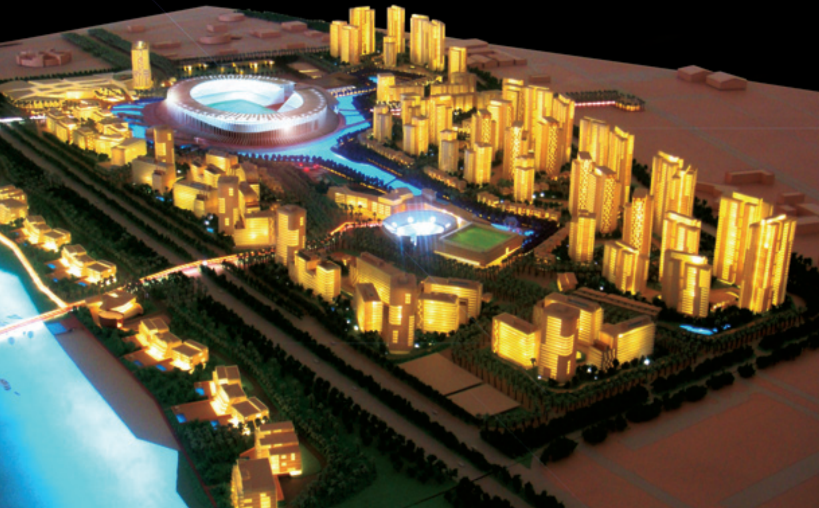
Integrated development in Abu Dhabi, UAE
