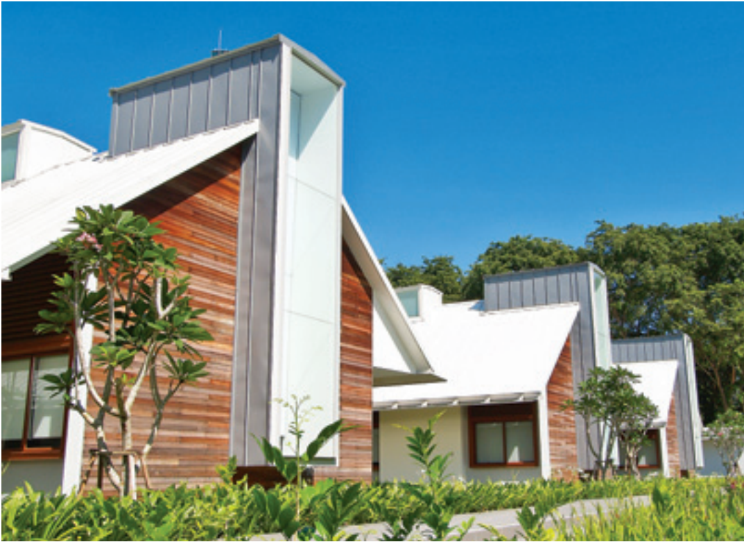
Ascott Centre for Excellence, Singapore – Ascott's new global hospitality training centre
