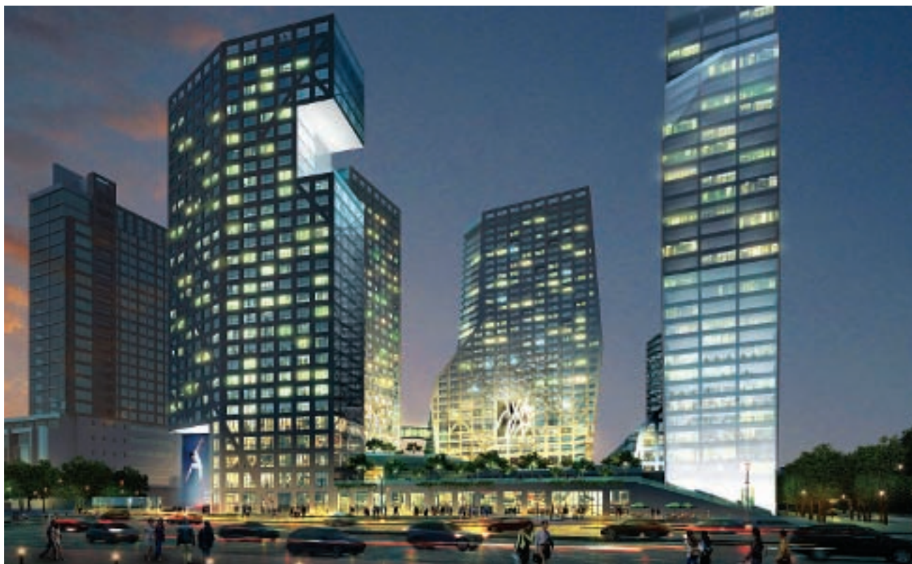
Construction is in progress for Raffles City Chengdu, one of CapitaLand's five Raffles City developments in China.
