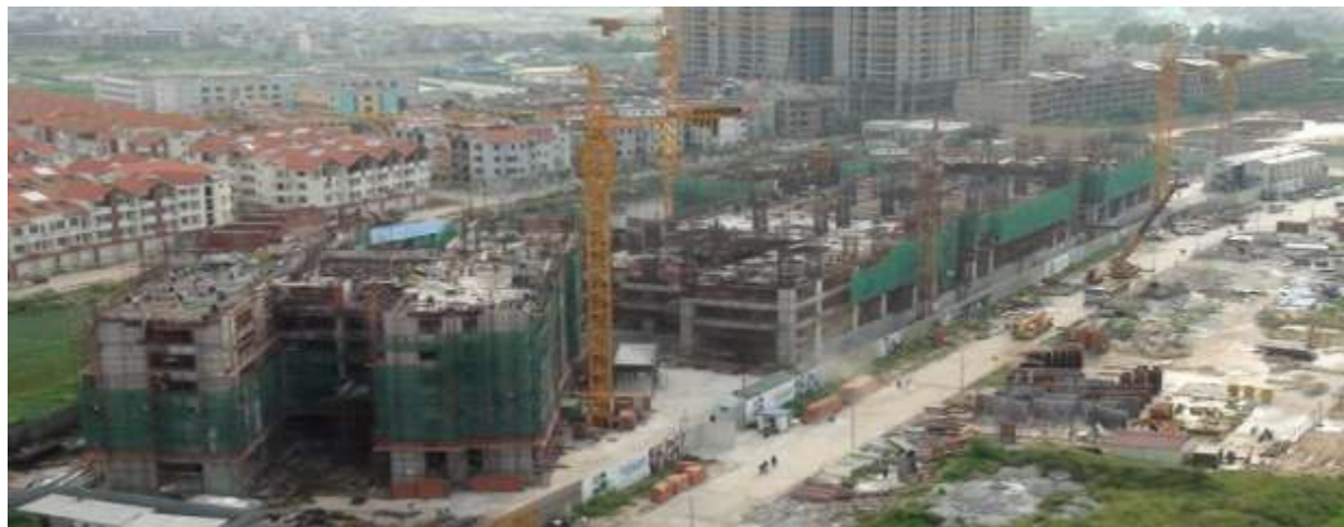
Construction of superstructure in progress
