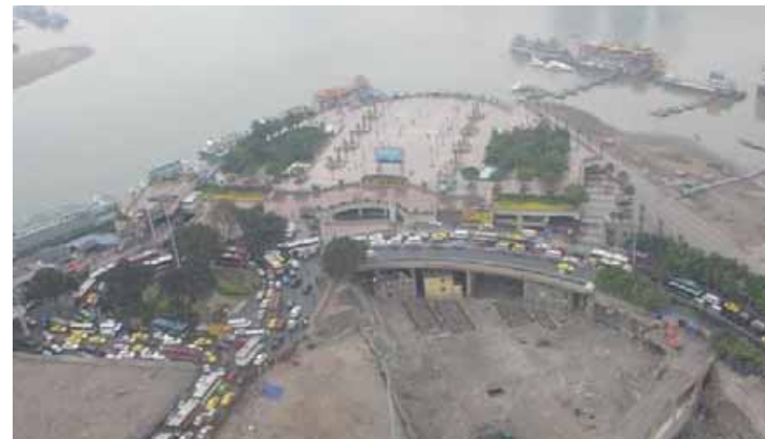
Site clearance in progress
