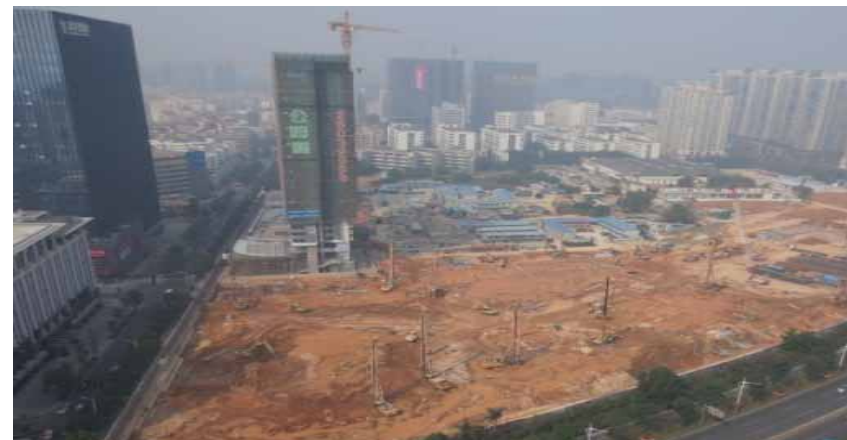
Excavation and shoring system in progress
