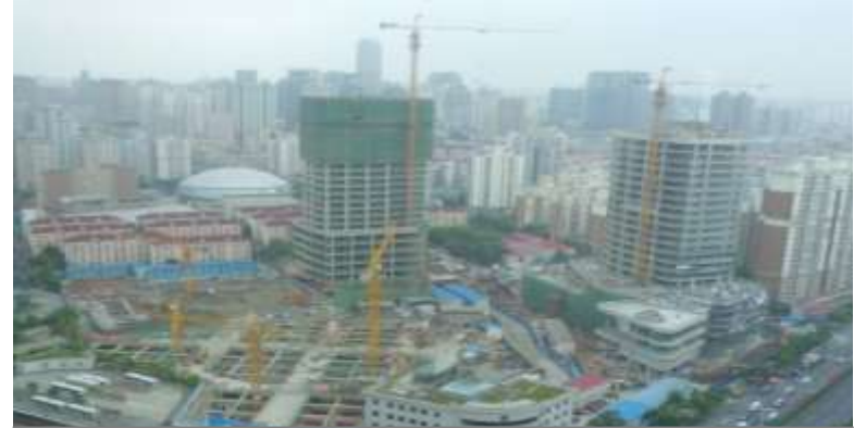
Structural Top-out for Tower 3
