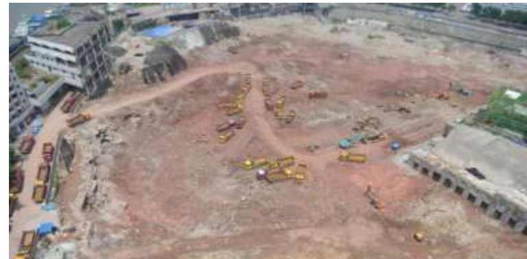
85% of Excavation and Lateral Support works completed
