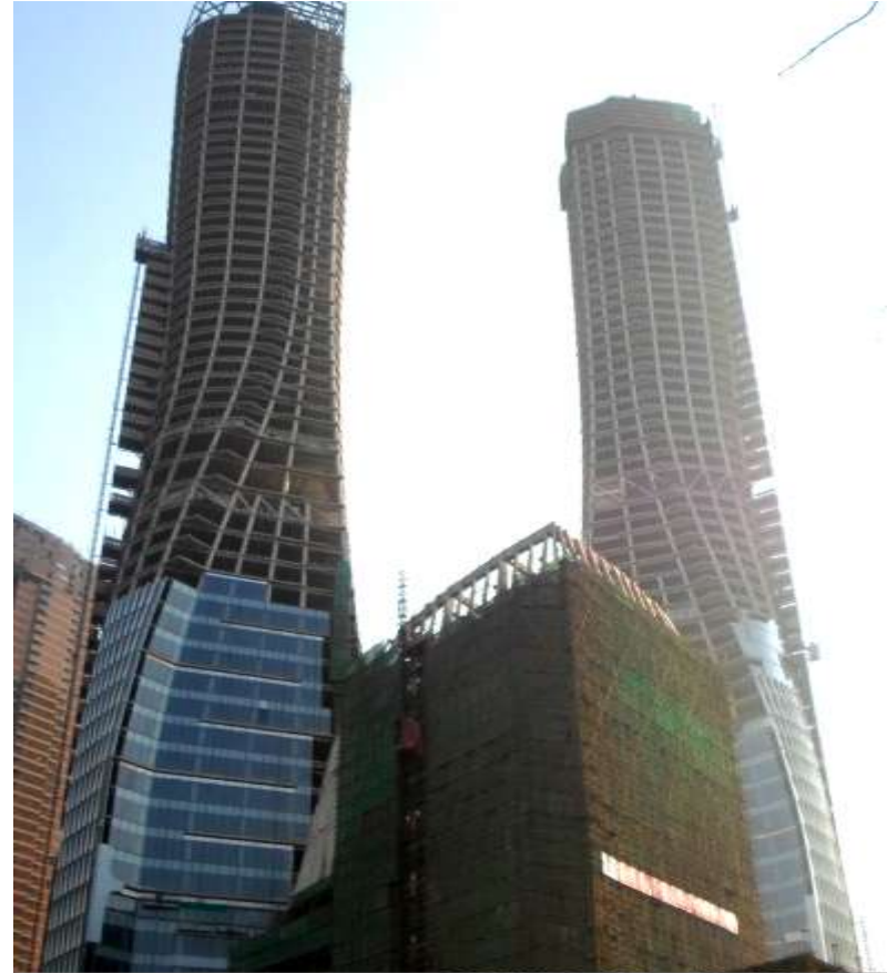
Curtain wall installation in progress
