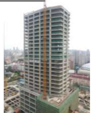
Structural Top-out for Tower 2
