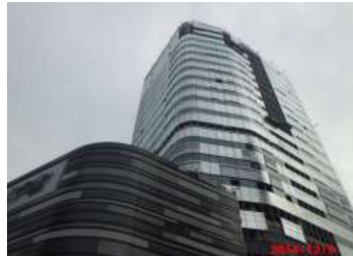
Curtain wall installation at West Podium & Tower 3 in progress
