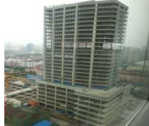
Structural completion for Tower 2
