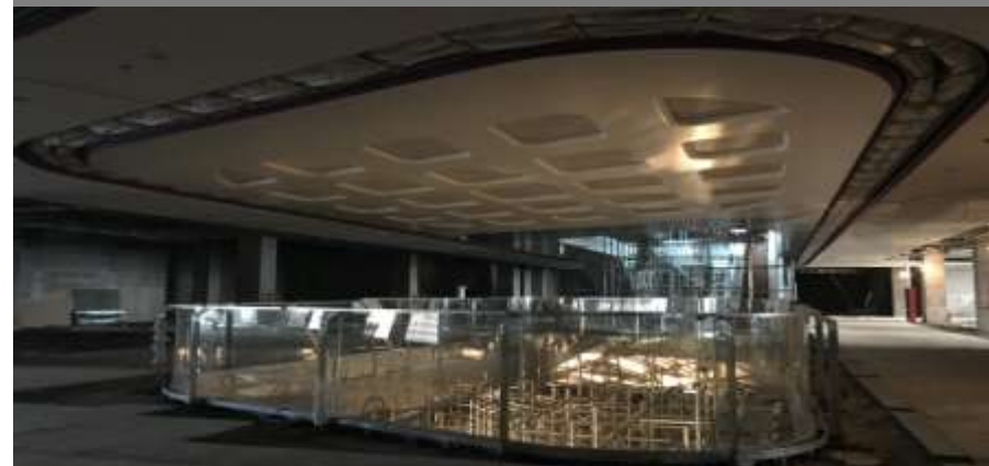
Mall Interior Works In Progress
