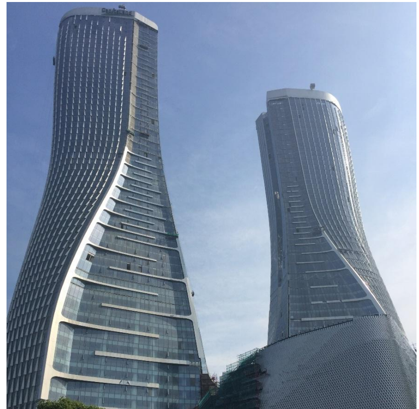
Curtain Wall Installation 95% Completed
