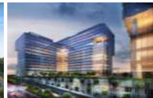
International Tech Park Pune, Kharadi
