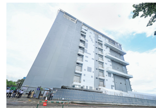
CIDCF acquired 20.2% interest in three data centres in India, including CapitaLand Data Centre Mumbai 01 (pictured).
