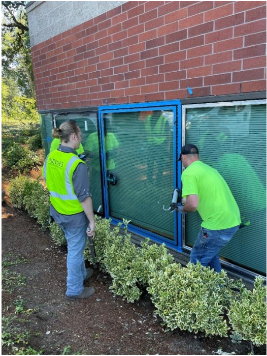
INOVUES insulating glass retrofit installation at one floor of Creekside 5
