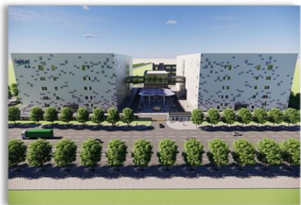
Two hyperscale data centre developments (CapitaLand China Data Centre Partners)
